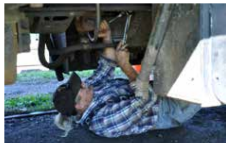
Lynn Butts installs new bolts in the coupler pocket.
